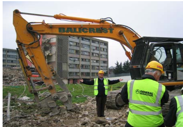
Former estate on Tanner Street undergoing demolition
